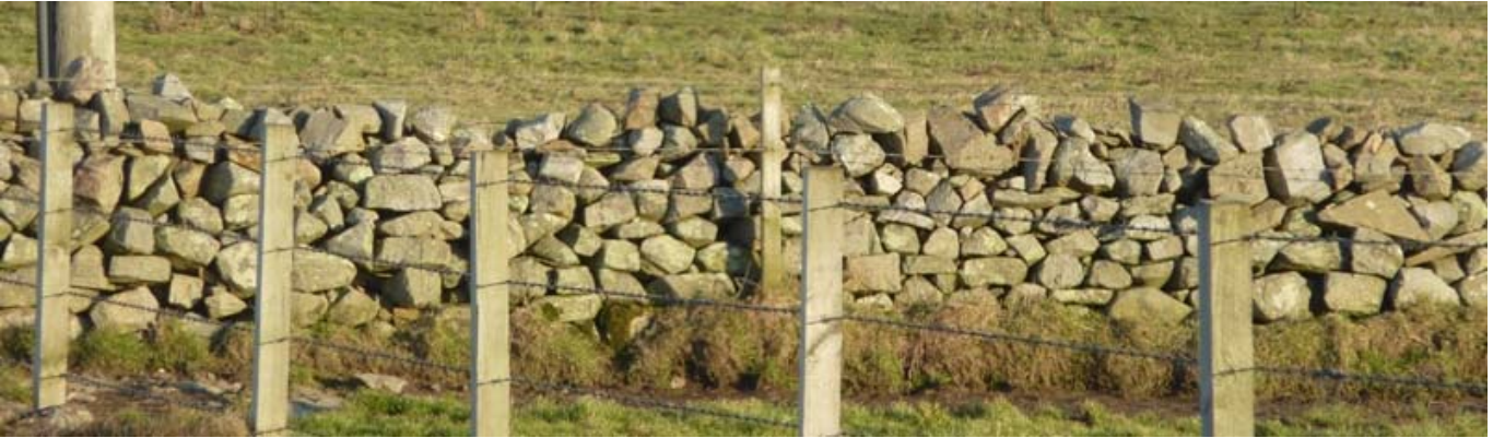
Traditional Stone Dyke near to development site
