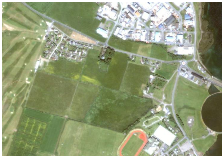
Fig 1: Aerial View of Site (prior to development of adjacent Council Housing site)
