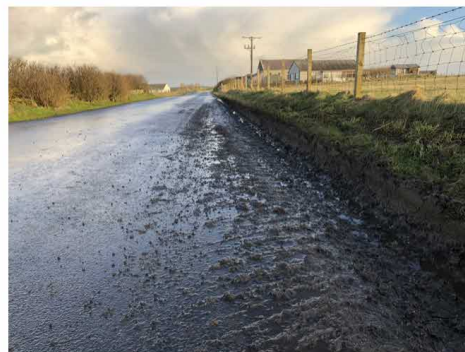
Agricultural vehicle damage on opposite sides of public road at application site
