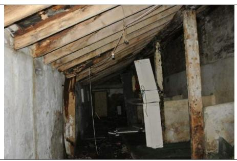
Figure 34: Interior of Building 7. Note staining of timber by water penetration. Photo: Tom Hunter
