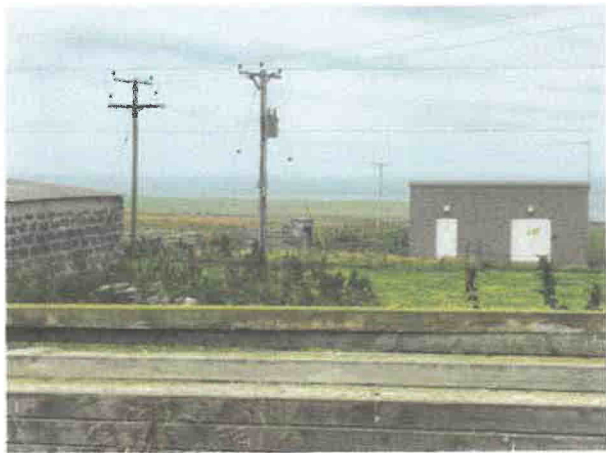
Photo 16 Wind turbine sub-station
