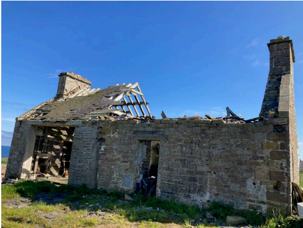
North elevation of farmhouse
