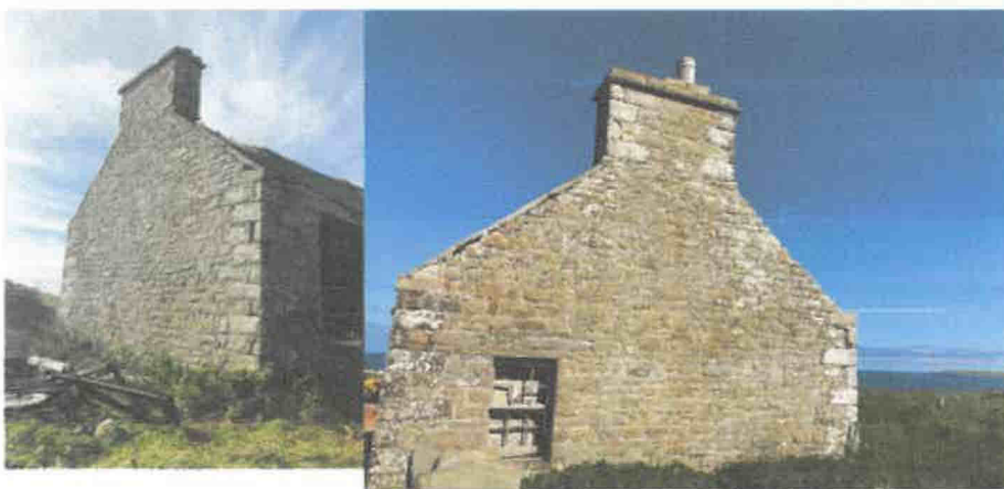
Photo 7 & 8 Gable ends of redundant farmhouse
