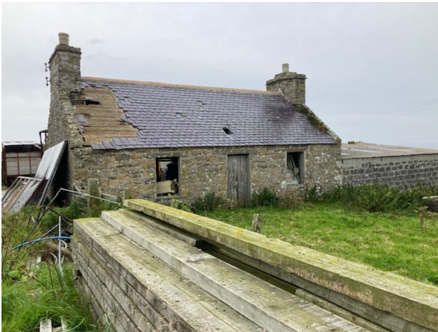
South elevation of bothy
