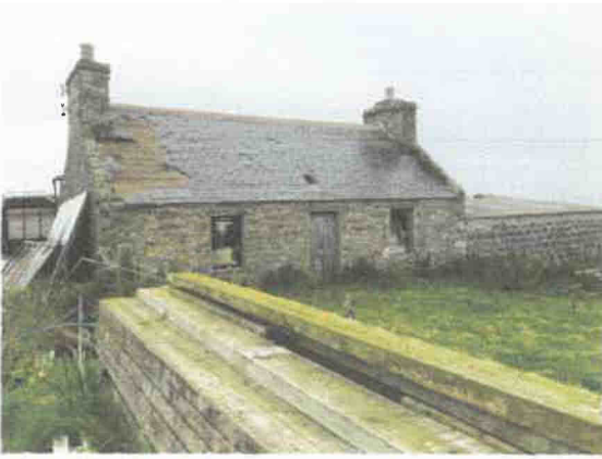
Photo 2 South elevation of redundant bothy.
