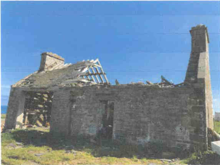
Photo 10 North elevation to farmhouse.
