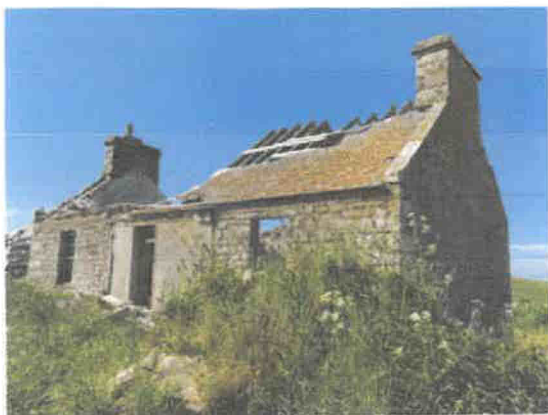
Photo 12 South elevation of former farmhouse
