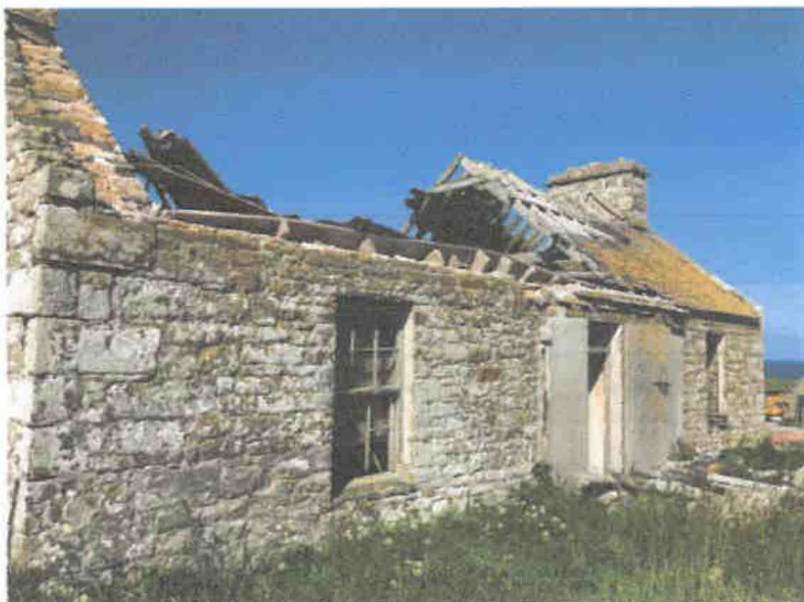
Photo 11 South elevation of former farmhouse
