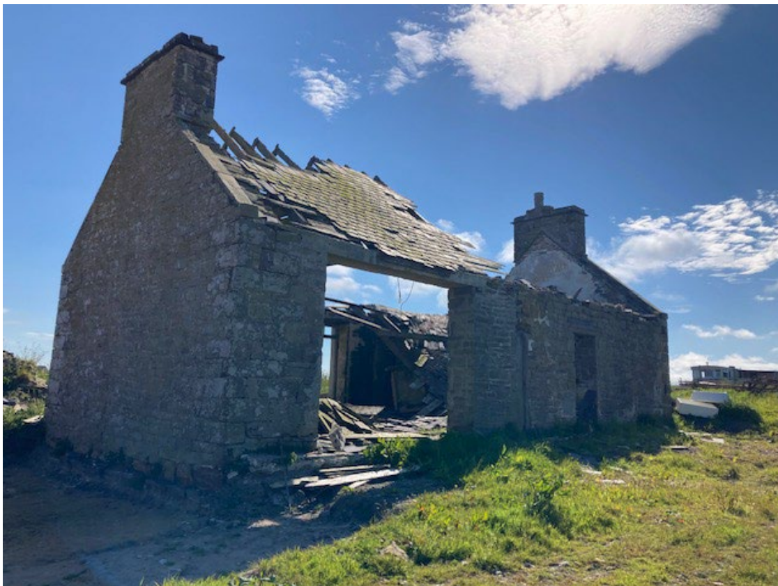
North elevation of farmhouse
