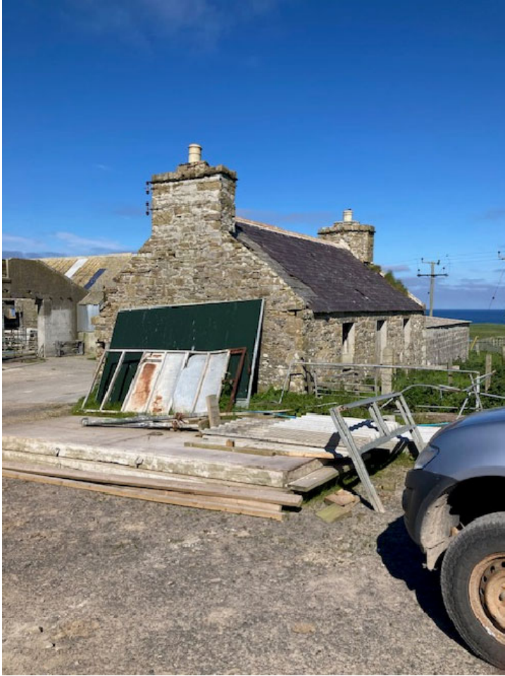
South elevation of Bothy
