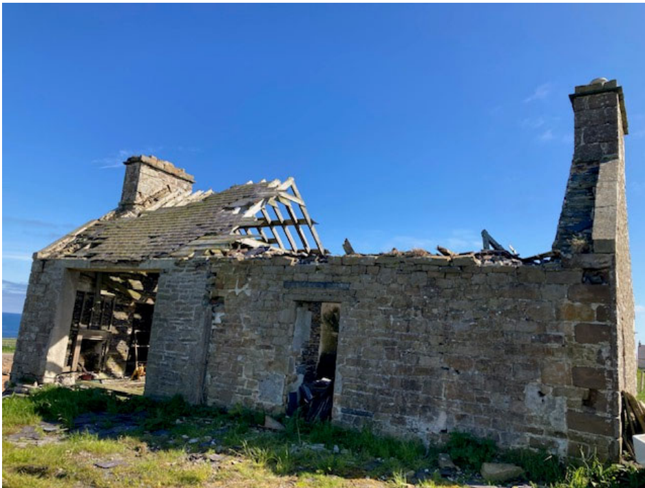
North elevation of farmhouse
