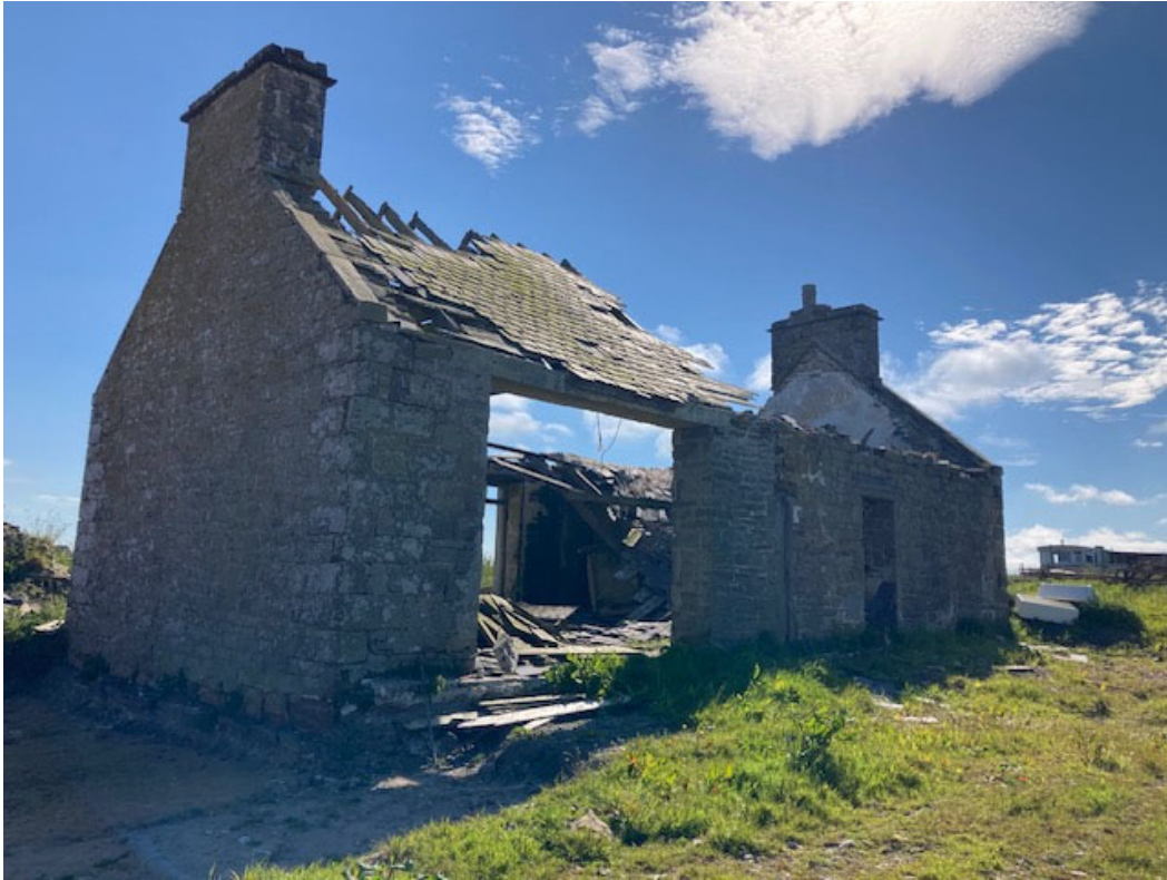
North elevation of farmhouse
