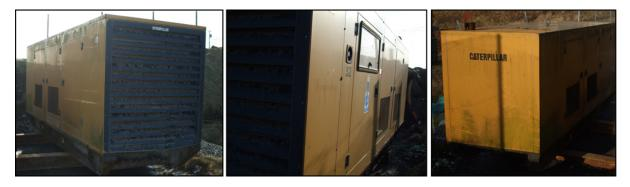
Caterpillar 3306B generator, 200kW, 400 v (3 phase), 250 KVA, manufactured 2003 with approximately 11249 working hours
