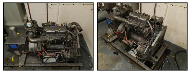
Newage/Stamford Type PC164E generator with Perkins Diesel Engine 3.152 series, 17.6kW, Serial Number: L7785/16 TO B.S. 5000/99, 380/415v (3 phase), 21.2 KVA, manufactured approx. 1987 with approximately 80 working hours.
