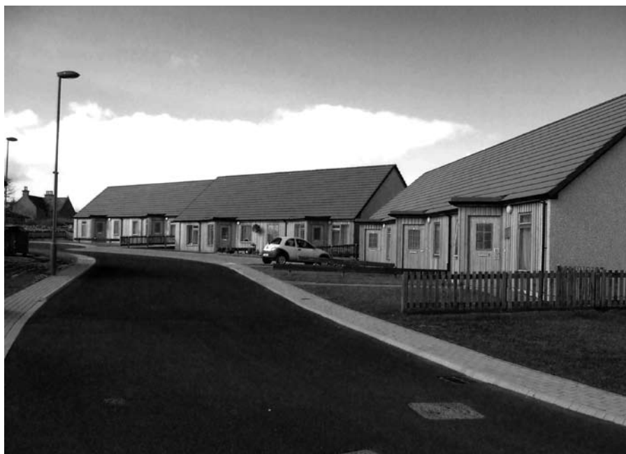
Sutherland Park, Kirkwall - New housing completed by Orkney Housing Association in 2007
